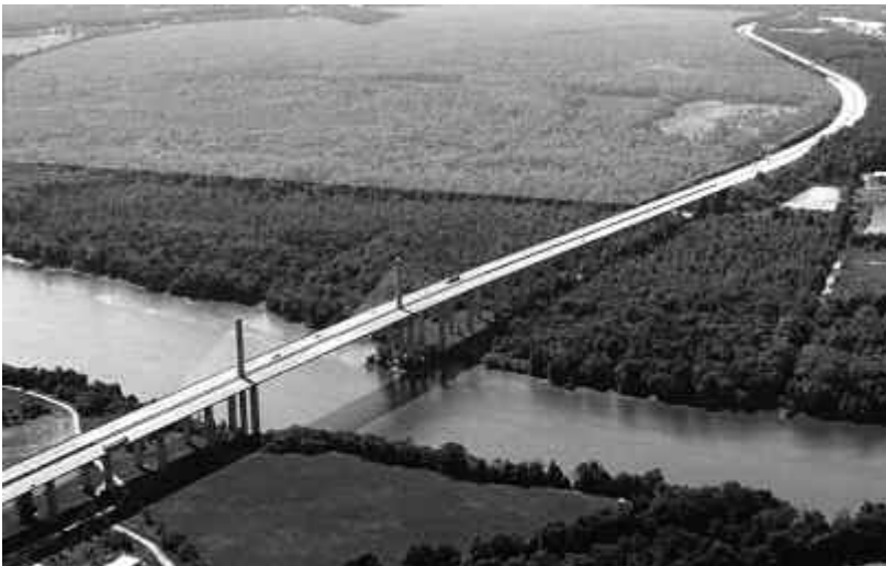
A view of Meadowville Technology Park (shaded area) looking southeast from the Varina-Enon Bridge over the James River.
