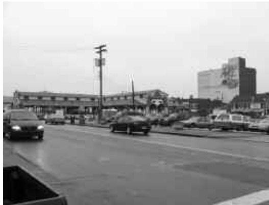
This view of Eastern Market shows development potential at the southern gateway.
