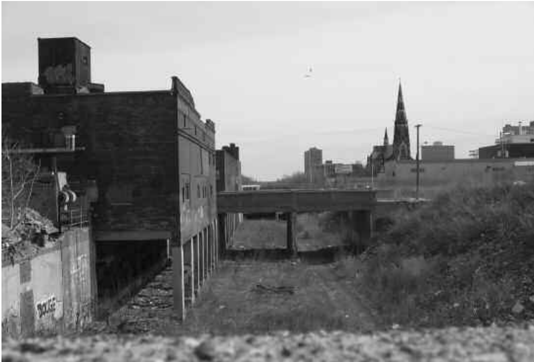
The Dequindre Cut is scheduled to be improved and will become part of the city's greenway infrastructure. This view shows the current condition of the rail right-of-way as it passes through the study area.
