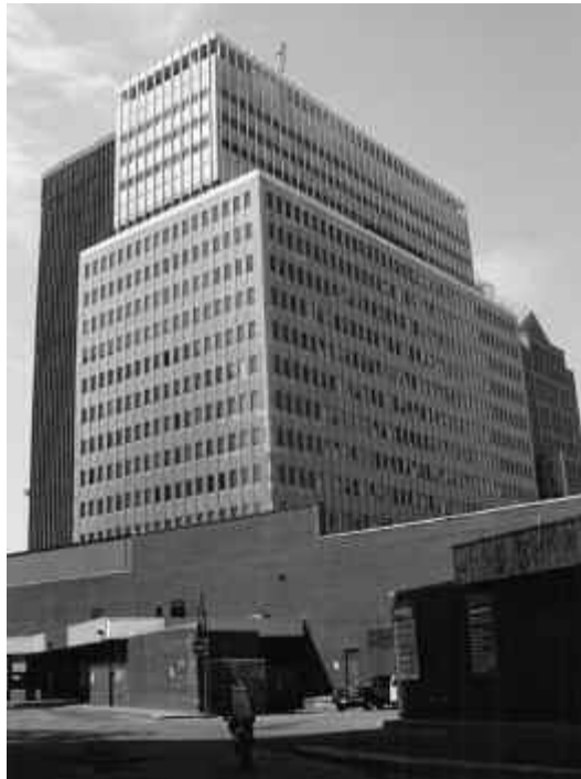
The Midtown office tower is mostly vacant but presents substantial problems with demolition.
