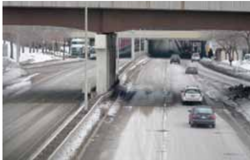
The Trench today divides the neighborhoods (right).
