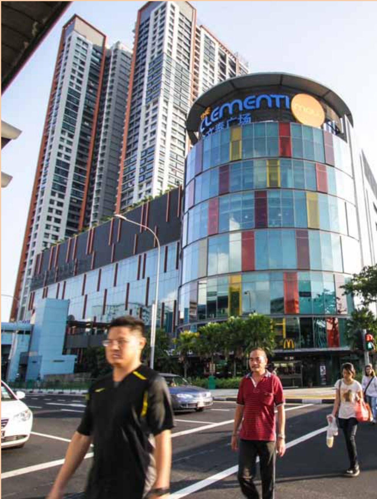
Clementi Mall is an example of a district node where a public mass transit station, bus interchange, retail outlets and a 40-storey public residential apartment are seamlessly integrated with one another. Photo courtesy of AECOM.
