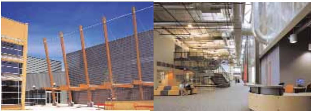
Forest City provided land and funding for construction of a "boutique" charter high school, the Denver School of Science and Technology, as part of the Stapleton redevelopment project outside Denver.
